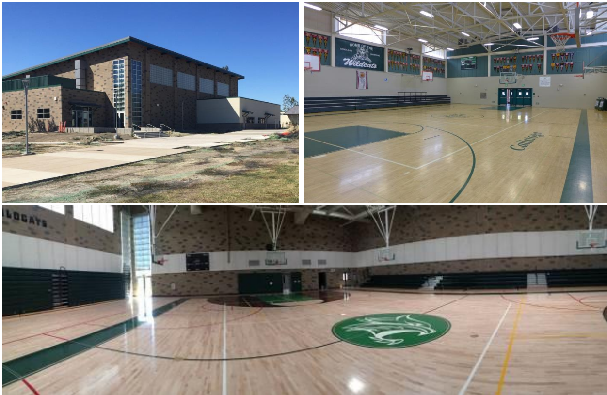
New gym facility at Calistoga Junior/Senior High, completed November 2013.
